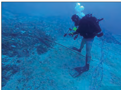
Construction Mechanic 2 nd Class Daniel Nichols (SCW/DV), Underwater Construction Team Two (UCT 2) Dive Detachment Alfa (CDDA), uses a cable tracker to identify and find deficiencies in an underwater cable at the PMRF.
