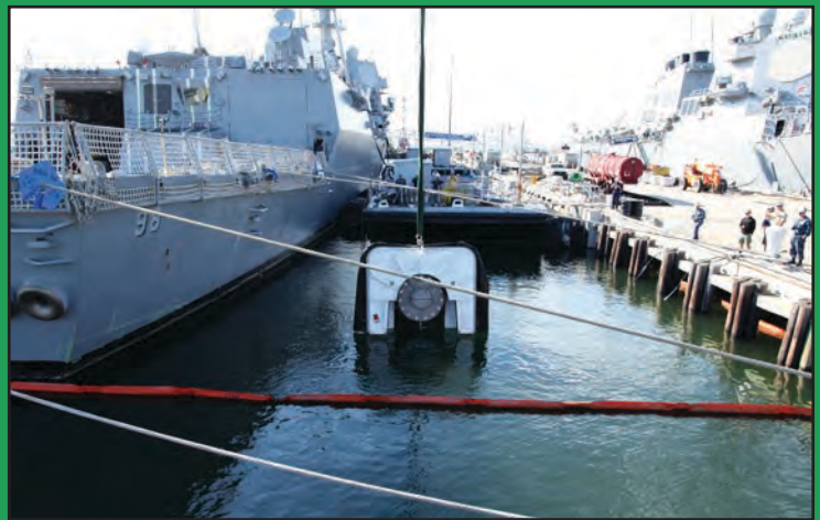
USS Forrest Sherman (DDG 98) hub and cofferdam are lifted out of the water pier after MARMC divers utilize the cofferdam to remove the hub underwater.
