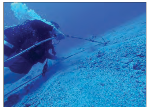
Builder 2 nd Class Justin Lieder (SCW/DV), Underwater Construction Team Two (UCT 2) Dive Detachment Alfa (CDDA), tracks an underwater cable and inspects it for damage at the PMRF.
